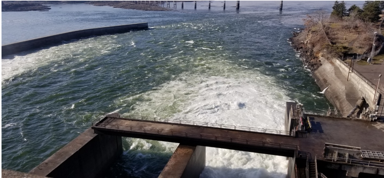
North entrance with spill gates 1,7,8 and 15Kcfs attraction water. 3/19/2019
